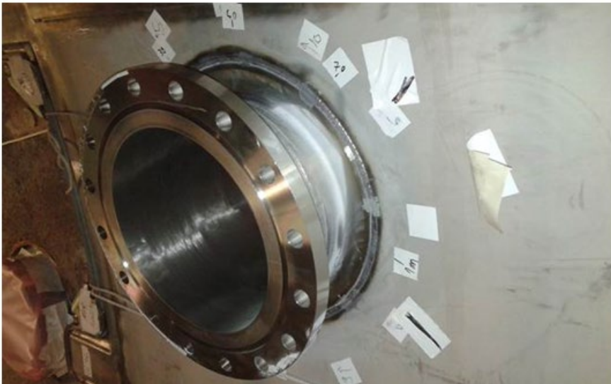
Full welding D9
