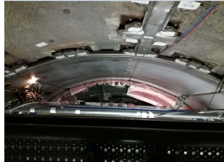
Welding and concreting of segment 2
