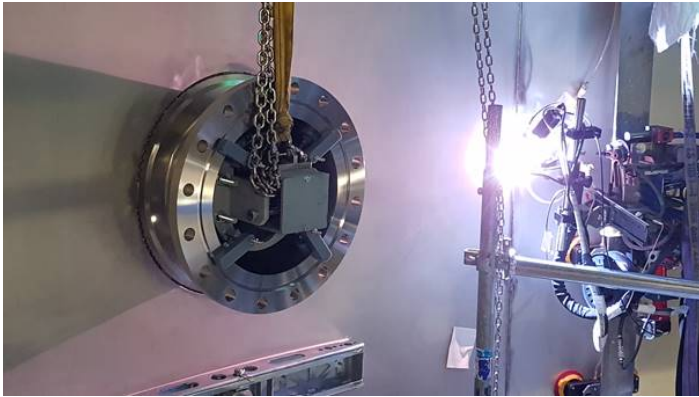
Sheet metal welding RER pool lining
