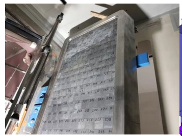
Installing lead panels
